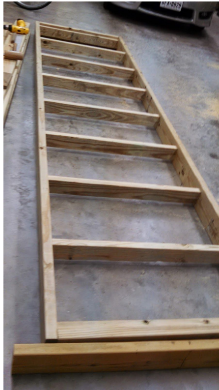
After adding stringers.
