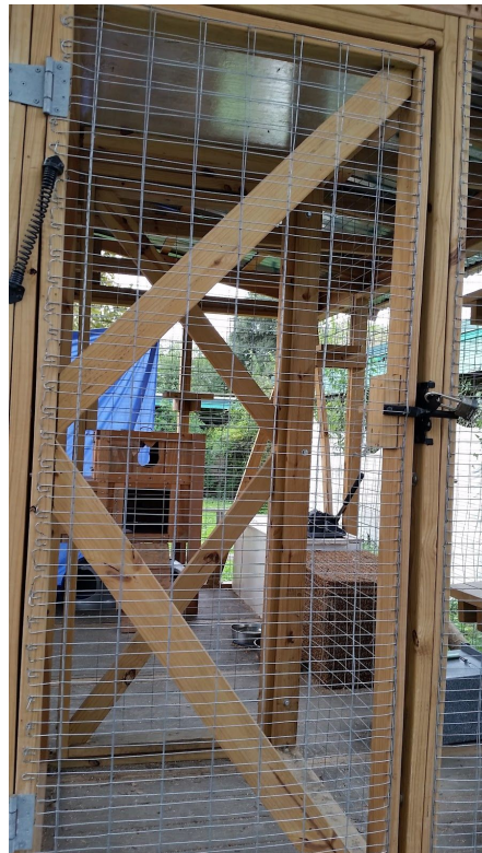
Photo showing the exterior door and supports, auto closer and latch.
