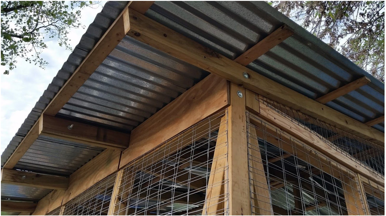
Photo showing corner, roofing panels, diagonal supports and blocking panels.
