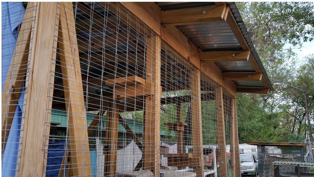
Photo showing roof overhang and connection details and platform attachment inside.
