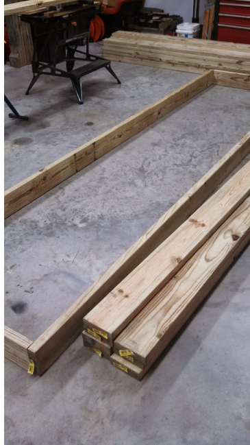
Photo showing 2 x 6 deck module prior to adding stringers
