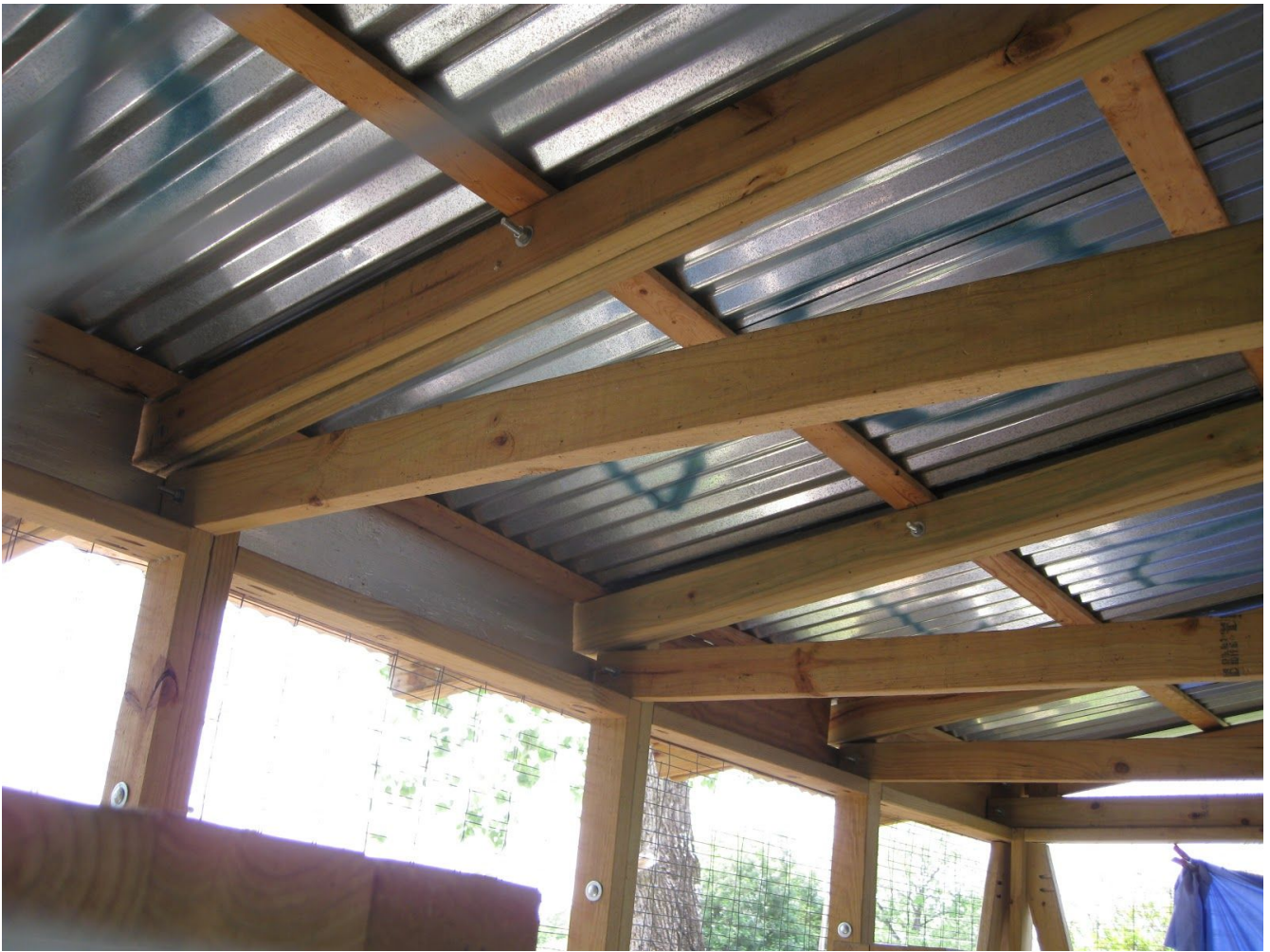
Interior shot showing truss, roof module, blocking wood, roofing and stringer details.
